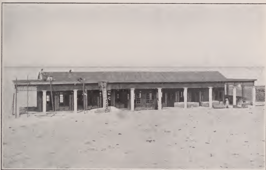
THE HOSPITAL AT KUWAIT IN COURSE OF CONSTRUCTION.
